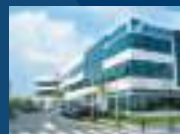
Daikin Holding USA
